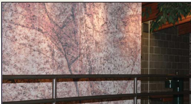
One-inch Tectum Panels on a C-20 mounting fixed the noise problem at Como Park Primate House.
